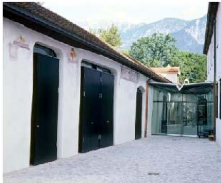
[Figure 4: Courtyard before and after restoration]
